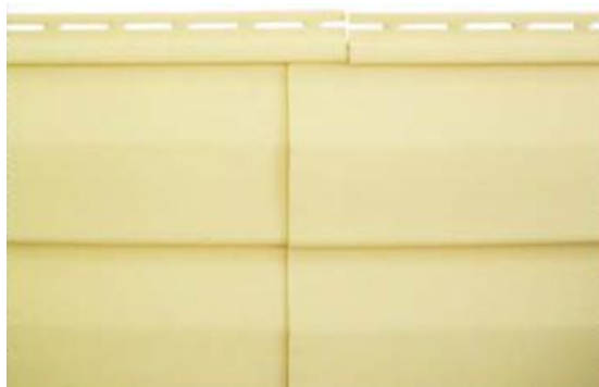
挂板搭接处理 siding lap processing the photo
